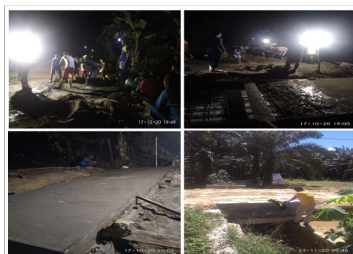
Figure 3. Cash for Work Activities in Mekar Mulya at Night
